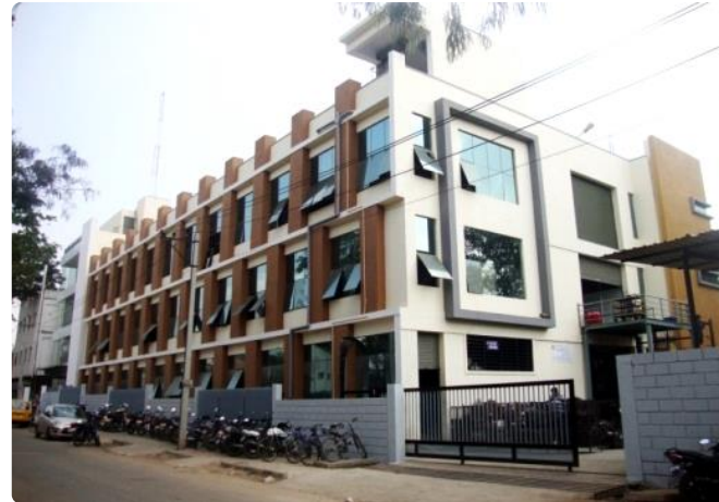
Dynamatic Hydraulics®, Unit II
