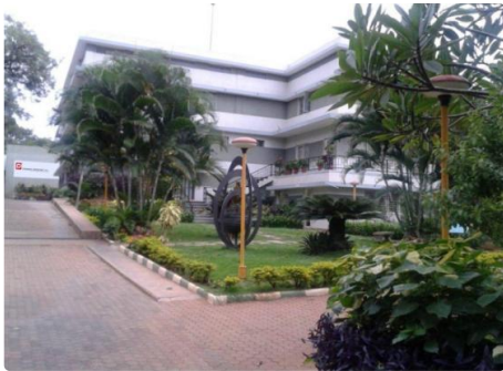
Dynamatic Hydraulics™, Unit I
