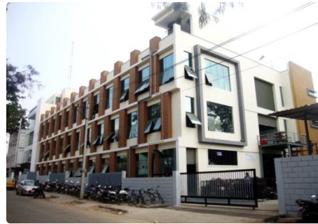
Dynamatic Hydraulics™, Unit II
